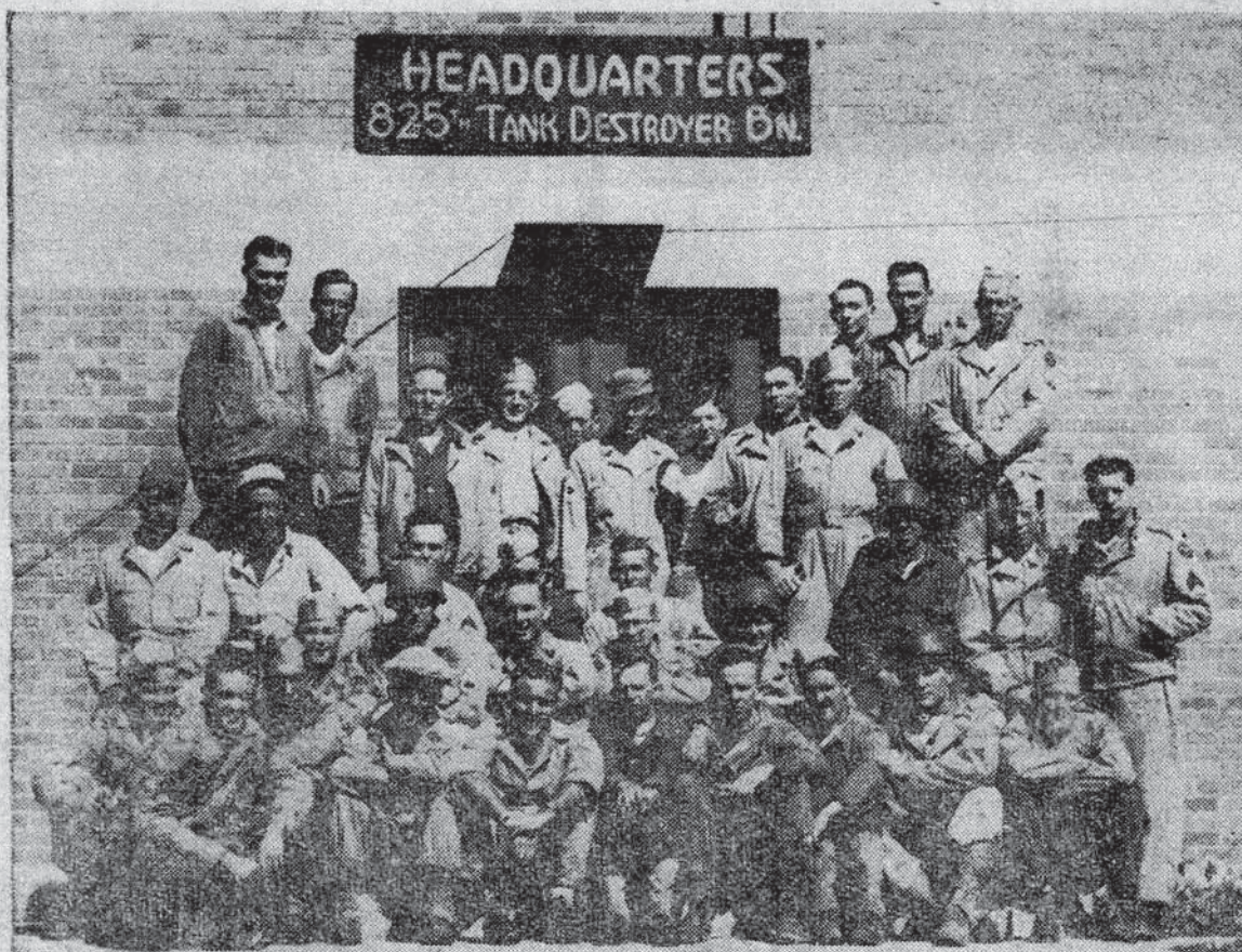
Men of the Battalion Headquarters Detachment stationed at Devils Lake. Clerks, supply, and motor maintenance personnel compose this group. Their tent-city on the corner of the county jail was one of the "sights" of Devils Lake, for 37 days.
